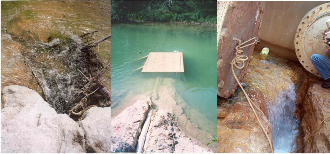
A series of pictures of Antioch Cave from left to right: Recharge into a pristine Antioch Cave entrance in Onion Creek; concrete vault and valve system build upon Antioch Cave which controls recharge; inside the vault.
