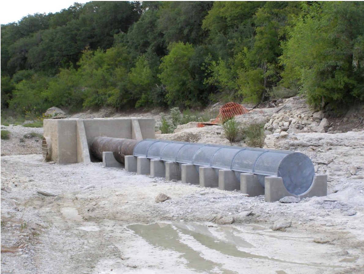
Antioch Cave vault with newly installed intake screen (Sept. 2008).
