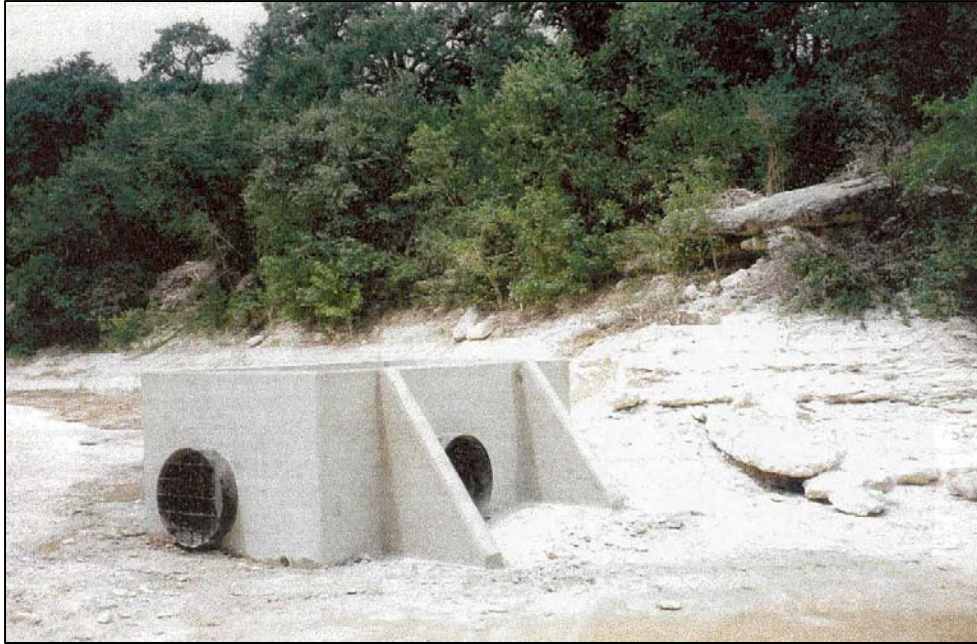
Figure 1-3. Photograph ca. 1997 showing the near-finished BMP vault over Antioch Cave; circular openings are 36 inches in diameter. (Photograph from Fieseler, 1998).
