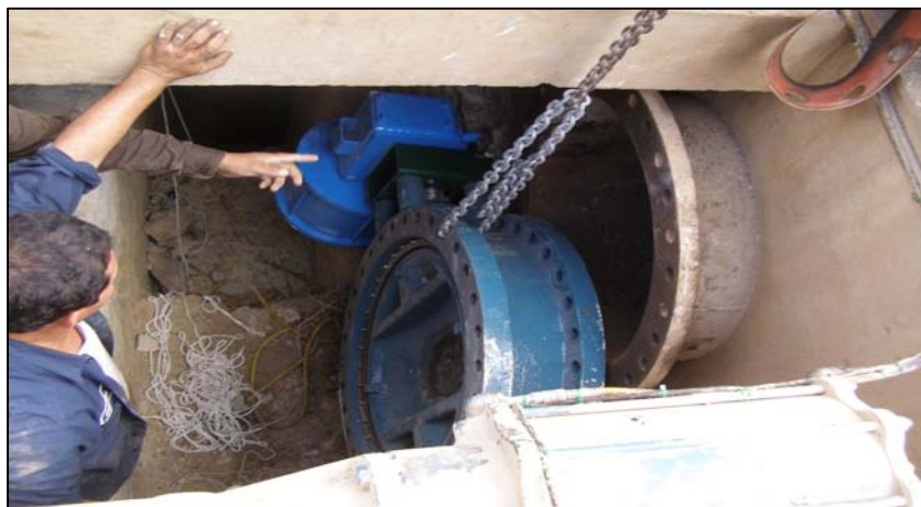
Figure 2-1. Installation of 2 nd valve (automated) on Antioch BMP.
