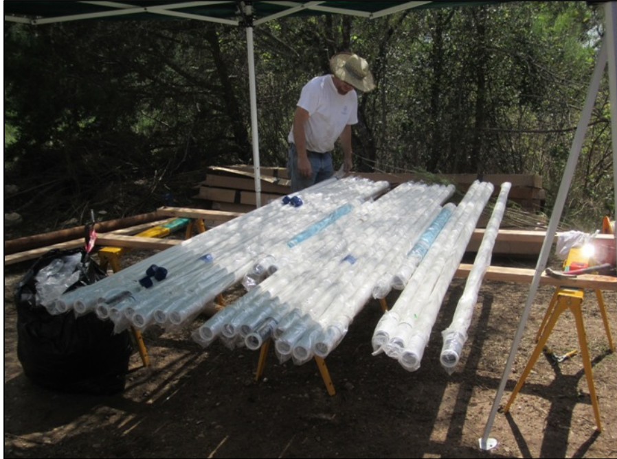
Figure 2-3. Photograph of layout of multiport monitor well components prior to installation.
