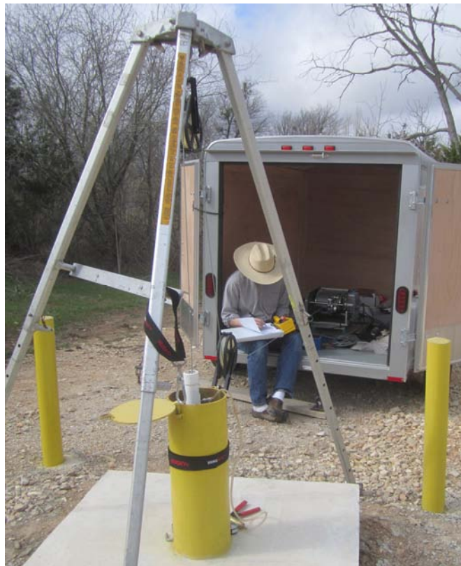
Figure 2-4. Photograph of the wellhead of the completed Antioch multiport monitor well during a sampling and water-level measurement event.
