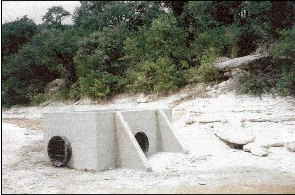
Photograph ca. 1997 showing the near-finished BMP vault over Antioch Cave; circular openings are 36 inches in diameter. (Photograph from Fieseler, 1998).
