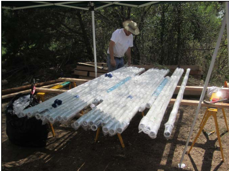
Photograph of layout of multiport monitor well components prior to installation.
