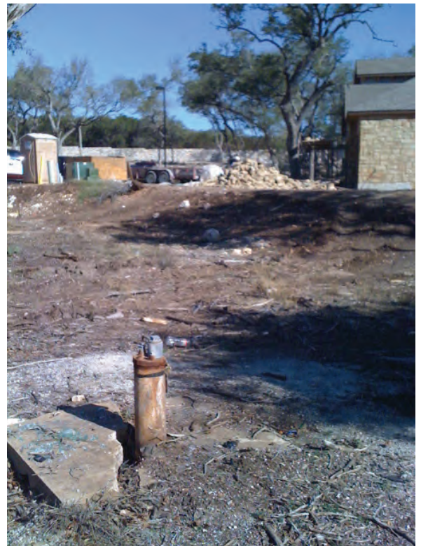
An unprotected, abandoned well with a cracked well head slab in a construction zone.
