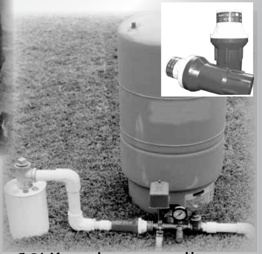
CSV1 on house well
