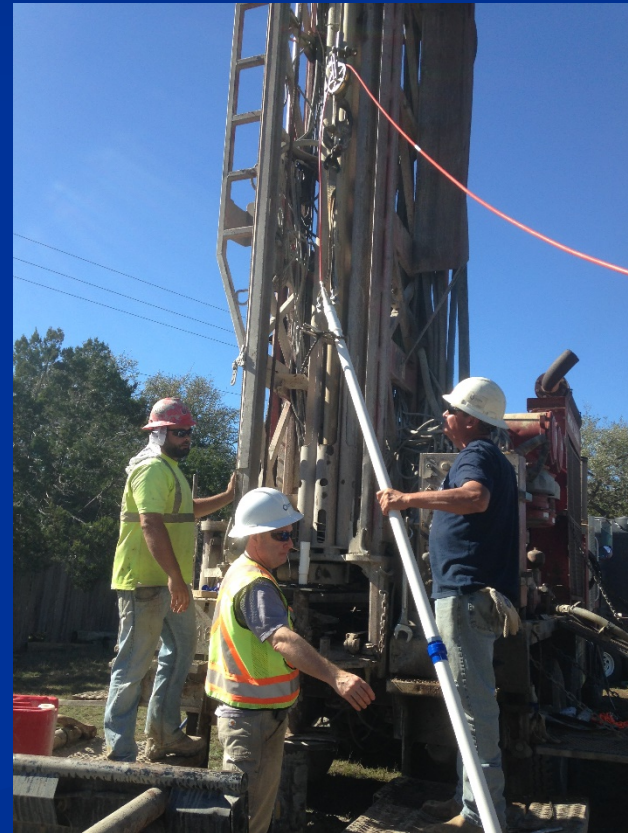
Installing into borehole
