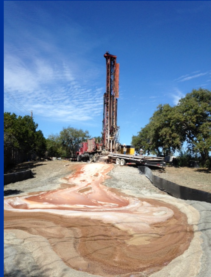
Travis County Multiport Monitor Well (2017)
