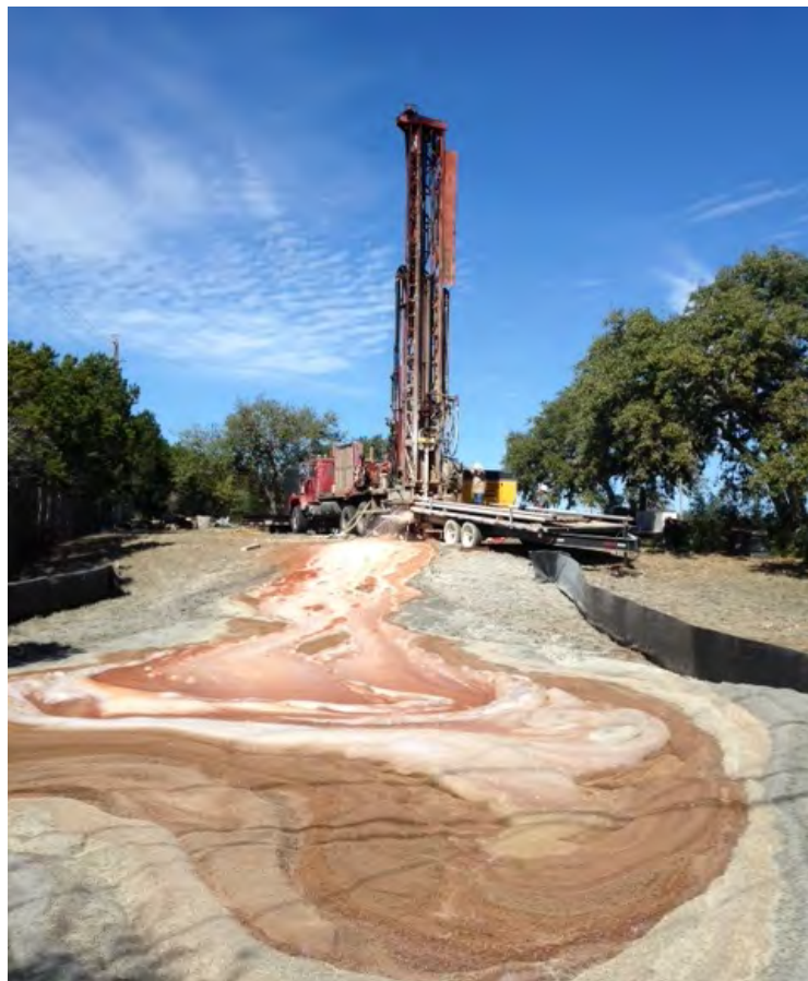
Figure 7. C&C Groundwater drilling a borehole for a multiport monitor well in Travis County, February, 2017.
