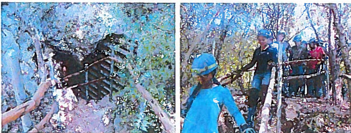
Figure 4. Addition of stairs, rails, and cave gate to LaCrosse Cave.
