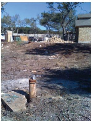
An unprotected, abandoned well with a cracked well head slab in a construction zone.
