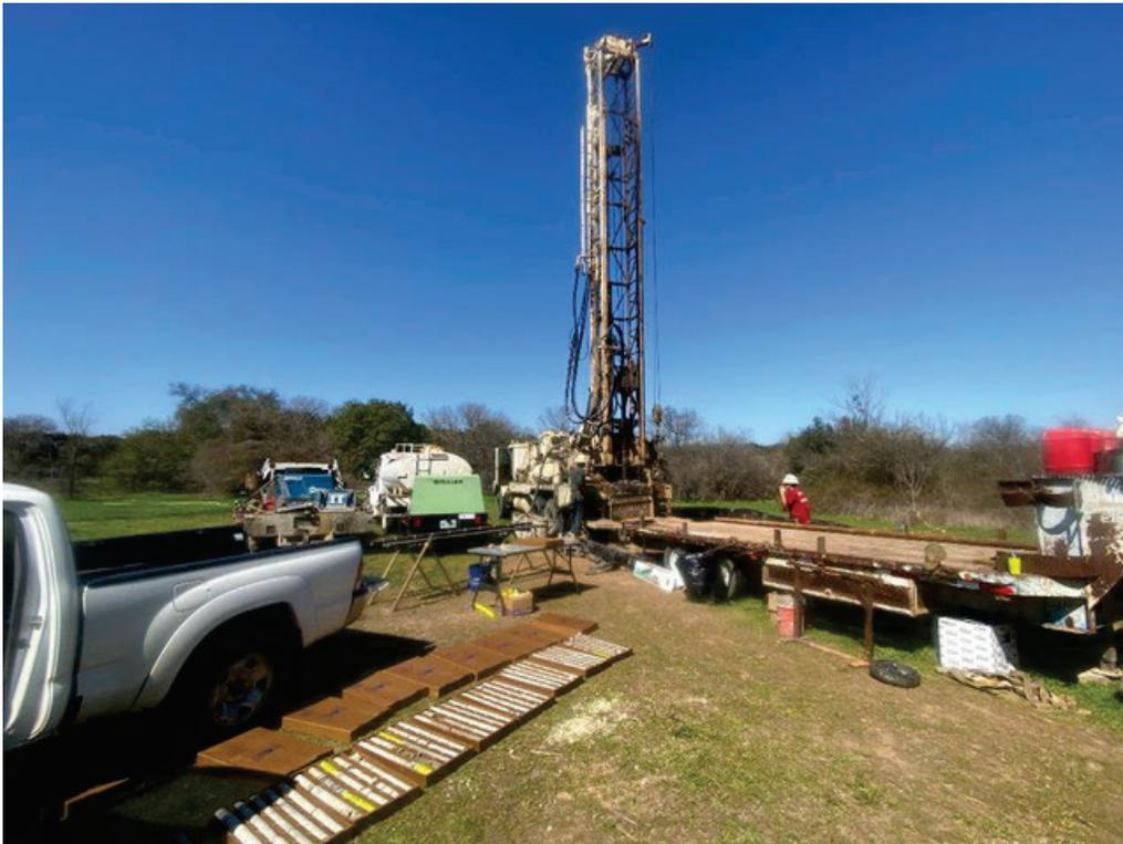
Figure 6. Photo of Barton Springs Multiport Well drill site. Core boxes filled with aquifer core samples can be seen in the foreground.
