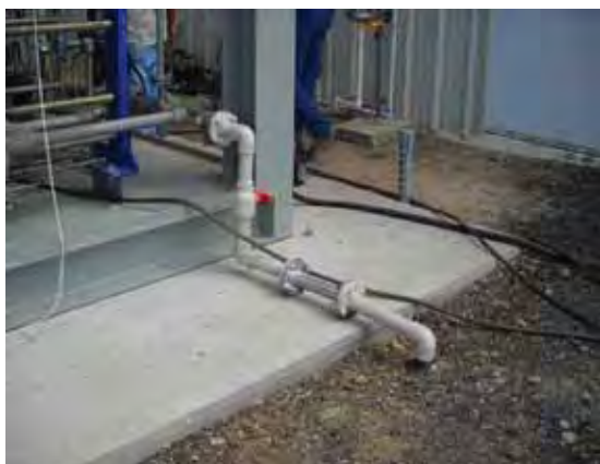
Figure 35. Brine Output Line to Brine Pit
