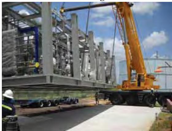
Figure 29. Skid Base Installation
