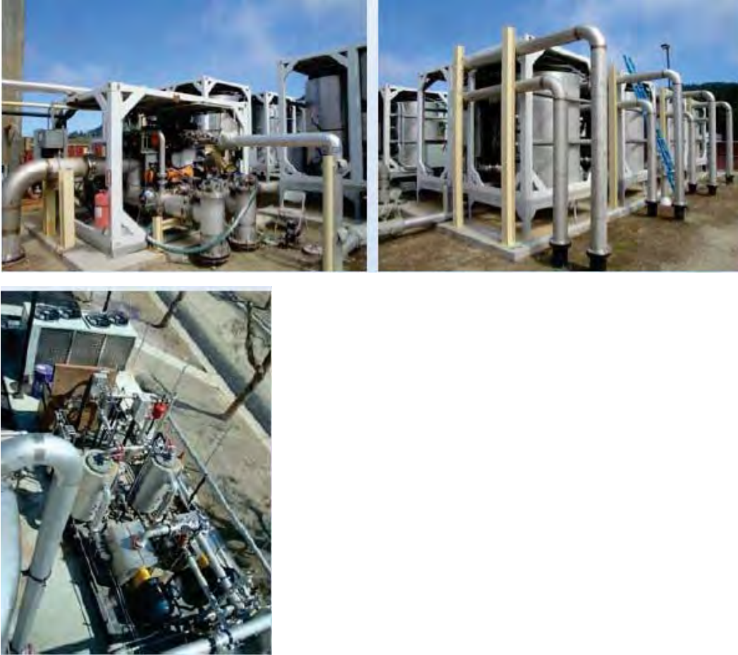
Figure 6.2 Gas Conditioning Skid
