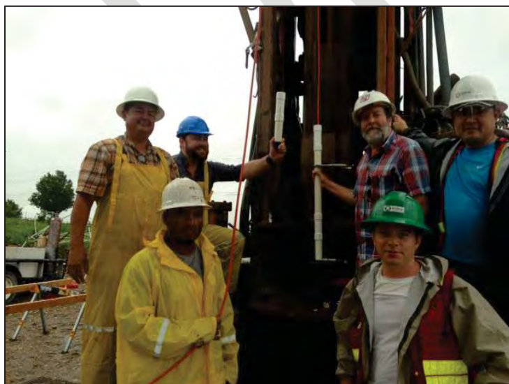
Photograph of the installation of the last Westbay casing piece in the multiport well. Photograph taken on 8/20/2016.
