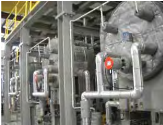
Figure 13. Installed Evaporators
