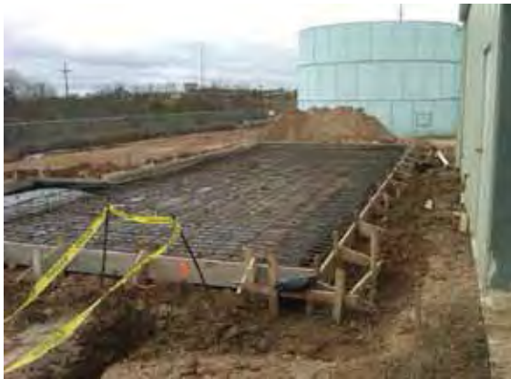
Figure 27. AdVE Skid Concrete Pad Framing
