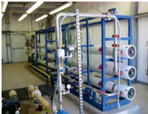
Figure 25. RO Plant Membrane Rack
