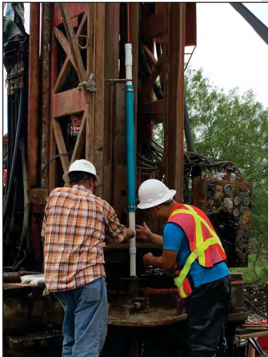
Figure 12. Photograph of assembly and testing of multiport coupling component. The coupling that connects the packer (blue, above) and the 10-ft casing section (white, below) is being pressure tested. Photo taken 8/20/2016.
