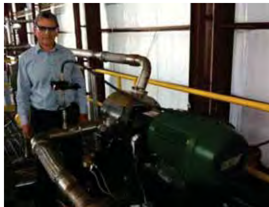
StarRotor Compressor Installed
