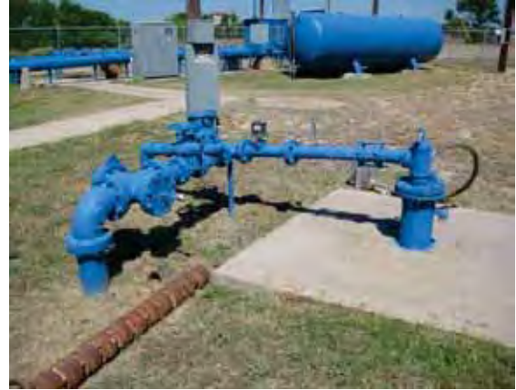
Figure 22. Santa Isabel Well (Note the old Submersible Pump on the Ground)
