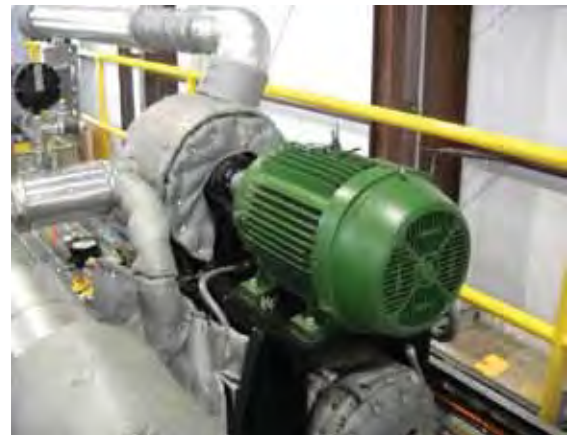
Figure 16. Star Rotor Compressor Installed on Top Platform
