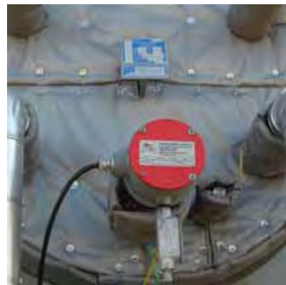
Figure 20. Start-up and Supplemental Heater in an Evaporator
