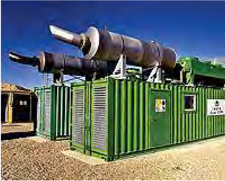
Figure 6.4 Self-Contained Generator Sets
