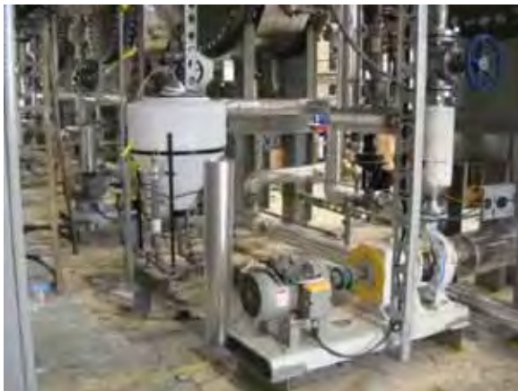
Figure 15. Brine Recirculation Pumps and Chemical Treatment Tank
