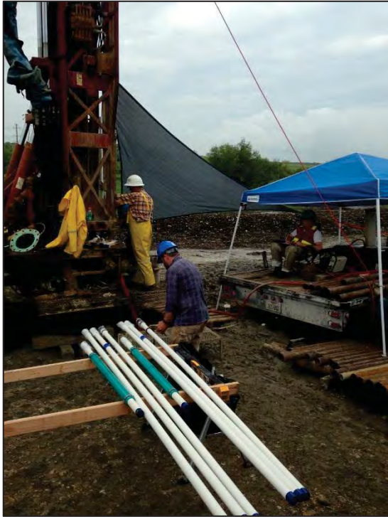
Figure 11. Multiport well components laid out for installation. Blue items are packers. Photo taken 8/20/2016.
