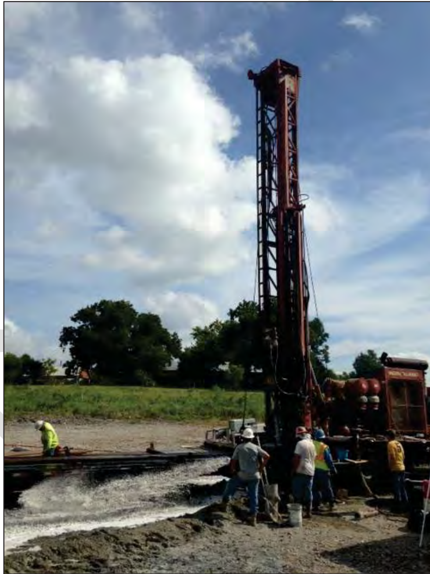
Figure 5. Drilling and development of the borehole for the multiport monitor well. Photo taken on 8/11/2016.
