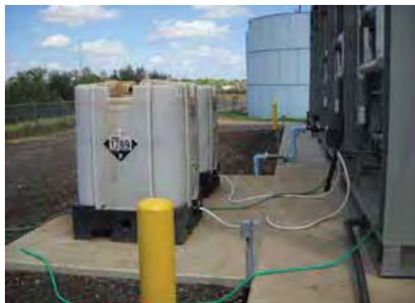
Figure 36. Chemical Tanks for Pre-Treatment of Well Water
