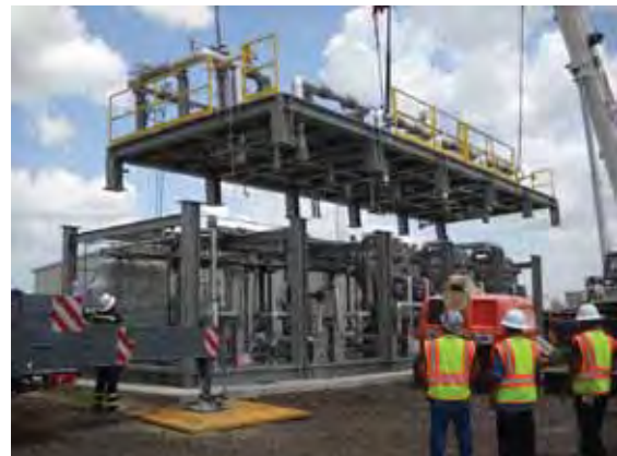
Figure 30. Skid Upper Platform Installation
