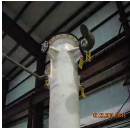
Figure 18. Carbon Dioxide Scrubber
