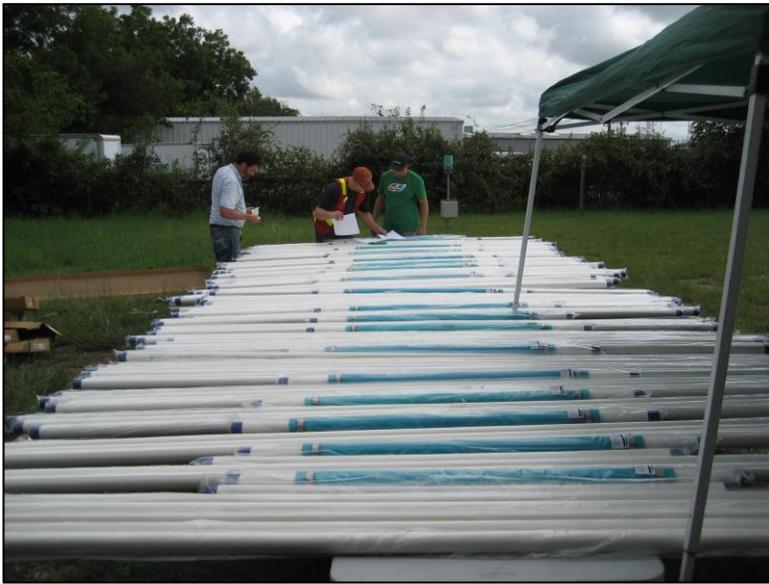
**Figure 5. Photograph showing layout and design of Westbay PVC casing system prior to installation. Blue sections are packers that separate zones.**
