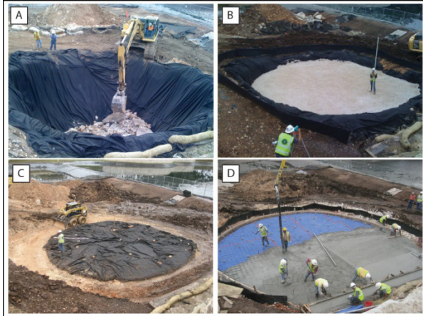
Figure 10. Photographs during sinkhole mitigation. A) Boulders and coarse fill and filter fabric; 5/2/12, B) graded cobble to gravel fill; 5/7/12, C) Gravel-filled sinkhole and filter fabric; 5/9/12, D) Reinforced concrete cap and blue vapor barrier; 5/10/12.
