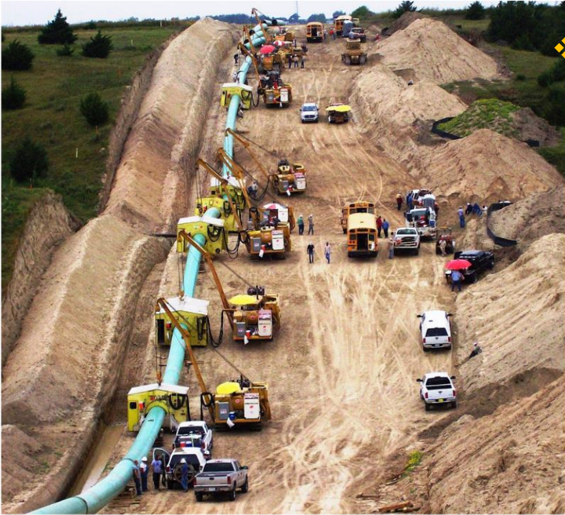
42' PIPELINE CONSTRUCTION IN THE NEBRASKA HILLS
