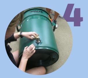
Place the second rubber washer over the faucet threads from inside. Place a locknut behind the rubber washer, then tighten faucet assembly. Apply silicone as needed. Let dry before use.
