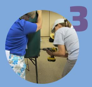
Drill a small hole near the base of the barrel. Check to ensure the drill bit matches the faucet size. Then thread a locknut and rubber washer onto the faucet. Insert assembly into the drilled hole.
