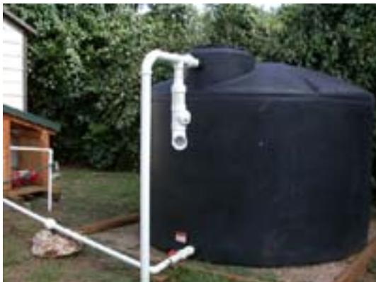
*The District collects water off a 640 sq. ft section of roof. The water is gravity-fed into a 1550-gallon black polyethylene tank, which becomes nearly full after a 4 in. rain. We chose this lightweight, dark-colored tank in order to prevent the growth of algae. It measures approximately 7'-6" in diameter by just under 6'-0" high.*
